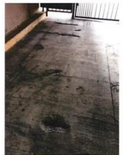
Figure J2: Spalling with exposed steel reinforcement at topside of garage deck.
