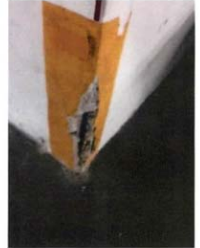
Figure J1: Typical cracking and spalling at parking garage columns
