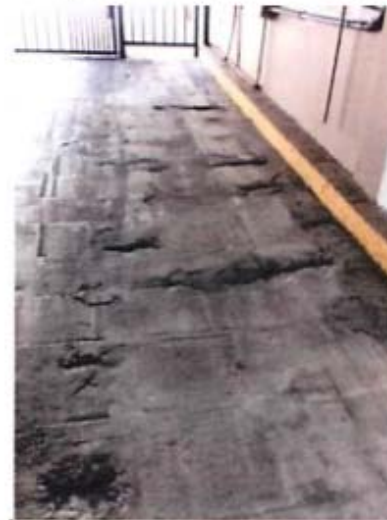
Figure J2: Spalling with exposed steel reinforcement at topside of garage deck.
