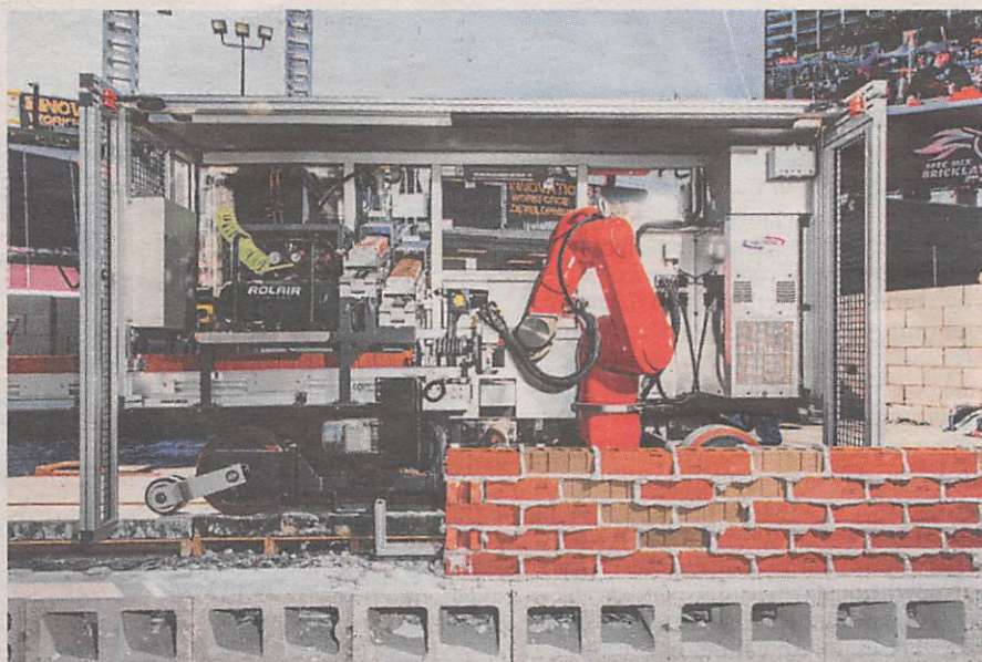
The SAM 100 (Semi-Automated Mason) is a bricklaying robot used for onsite masonry construction.
