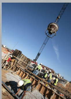
Skanska built this new wastewater treatment facility in Douglas County, Georgia.
